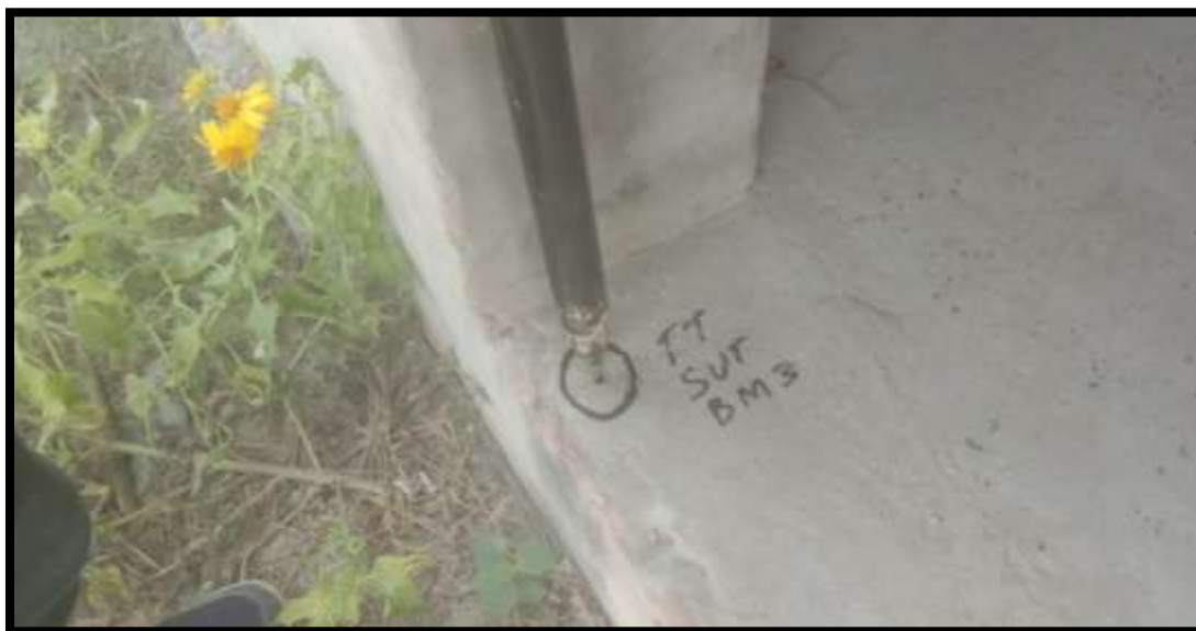
PHOTOGRAPH 6: Temporary benchmark creation in Sutlej River, Tarn Taran.
